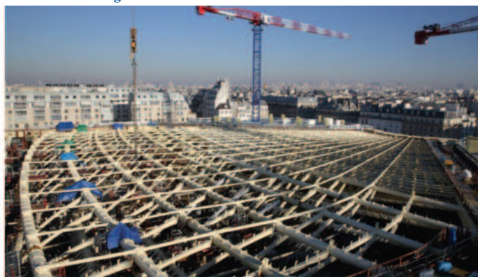
Figure 4 Phase de chantier (©H.Peter)
